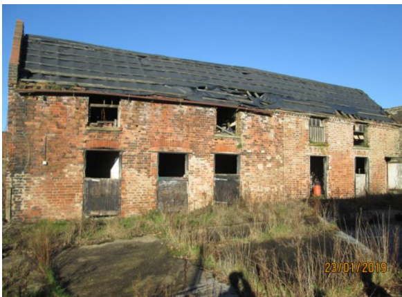
Front elevation of barn to be House 3.
