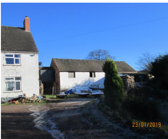
Front elevation of barn to be House 5.
