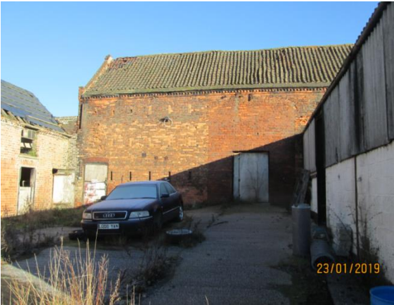
Front elevation of barn to be House 2.
